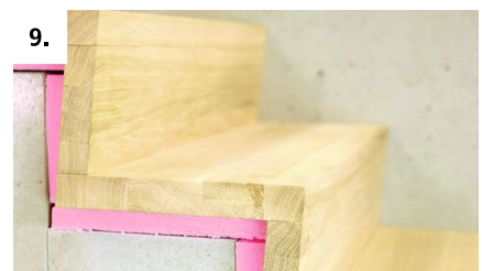
9. The folded plate staircase is finished.
