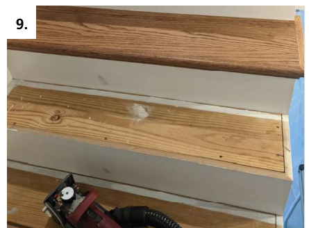
9. Tread is glued securely with no visible fasteners
