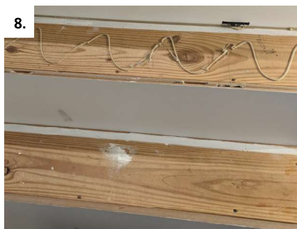
8. Install Tenso connectors and apply PL adhesive to rough framing and underside of tread
