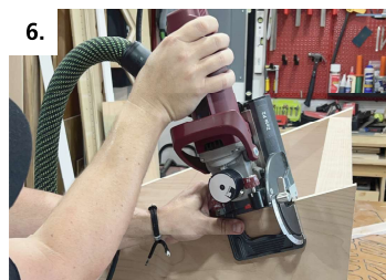
6. Machine slots in edge of hood frame uprights
