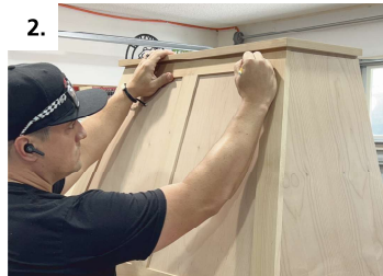
2. Transfer marks from front access panel to upper unit
