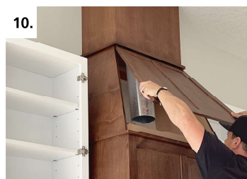
10. Slide top of access panel into place
